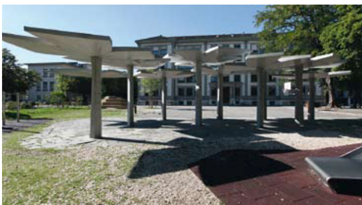
▲ FIG. 1 St. Johann school building, Basel. // ABB. 1 Schulhaus St. Johann, Basel.
