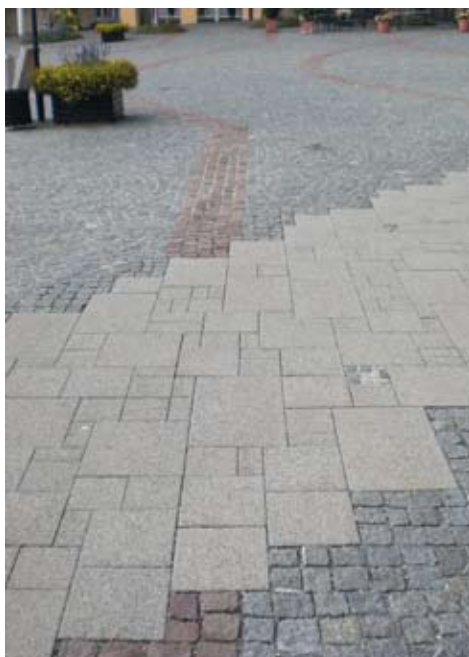
▲ FIG. 3 Successful companionship between concrete and granite pavement. // ABB. 3 Gelingendes Nebeneinander von Beton- und Granitpflaster.
