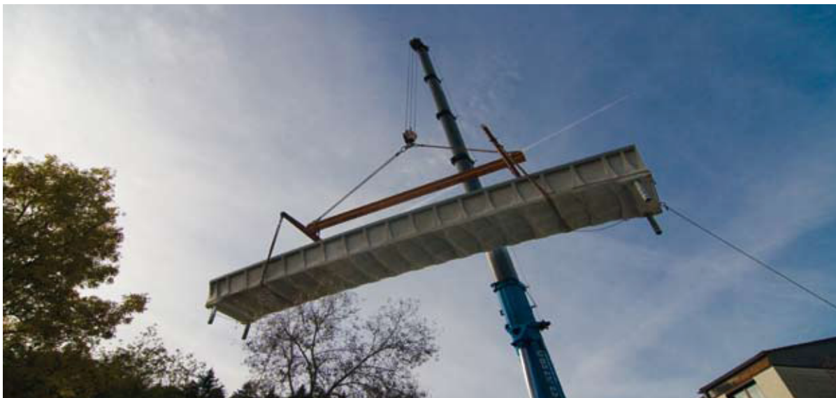
► FIG. 1 Textile-reinforced concrete bridge over the Rottach river in Kempten during assembly (photo by Ulrich van Stipriaan). //
