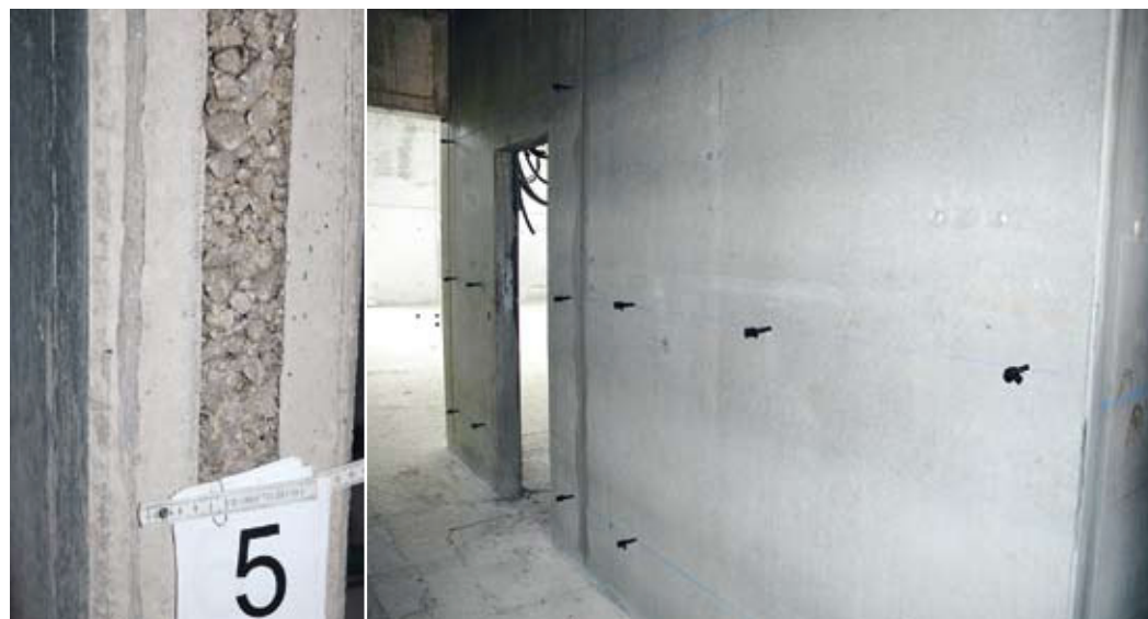
▼ FIG. 2 Grid of grouting packers. // ABB. 2 Raster der Bohrpacker.
