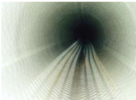
▲ FIG. 3 TROLINING® SelfCleaning System in installed condition [5]. // ABB. 3 Einbauzustand TROLINING® SelfCleaning System [5].
