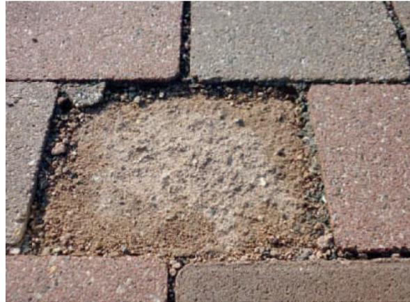
→ 1 Partially scaled facing layer of a concrete paver
