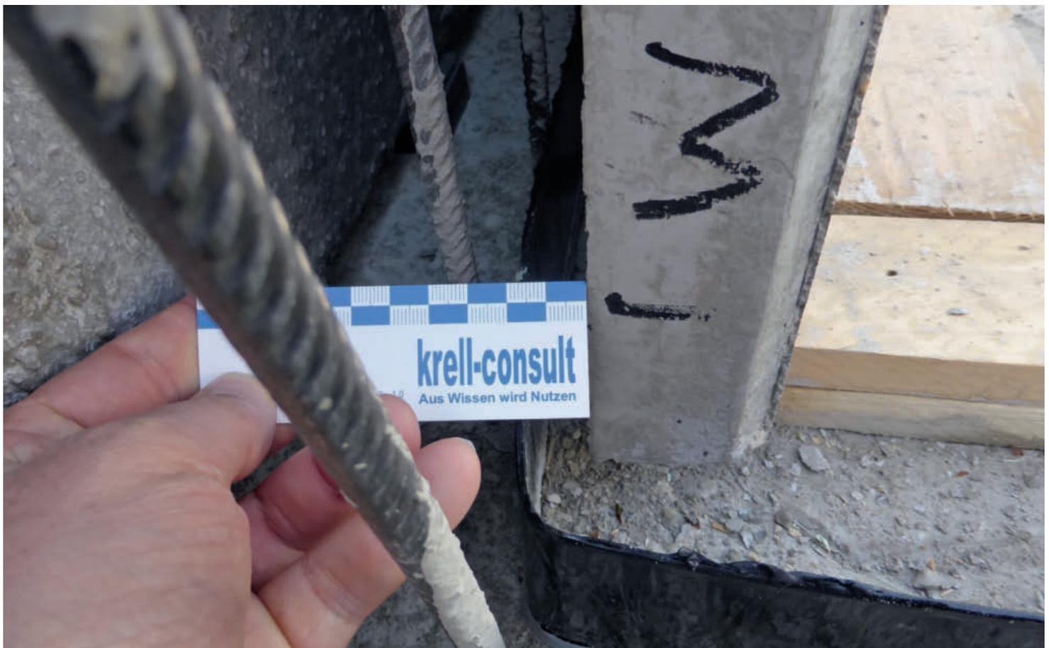
→ The space between joint sealing strip and reinforcement as well as the inner leaf of the double wall shall be at least 2 cm
