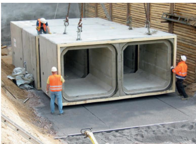
→ Sewer construction site using box culverts made of reinforced concrete
