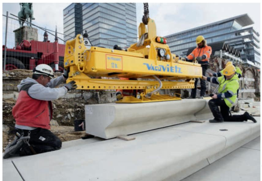
→ Rhine Boulevard – erection of a step
