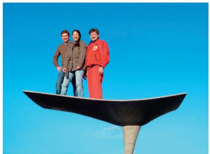
→ Roof shell Parapluie d= 25-30mm
