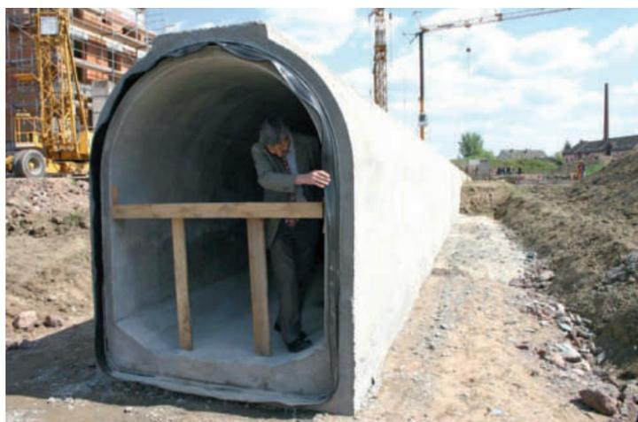
→ 3 Accessible pipeline for the accommodation of different systems within the network
